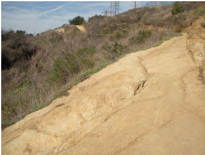
Realign and restore eroded trail segments on top of ridge.
